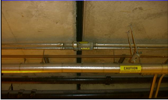
Building Expansion Joint
